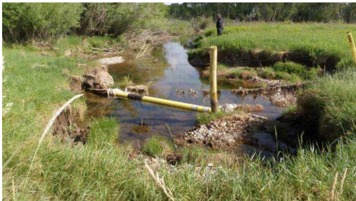
Conoco Phillips Glacier Pipeline at Belt Creek (Remediated)
