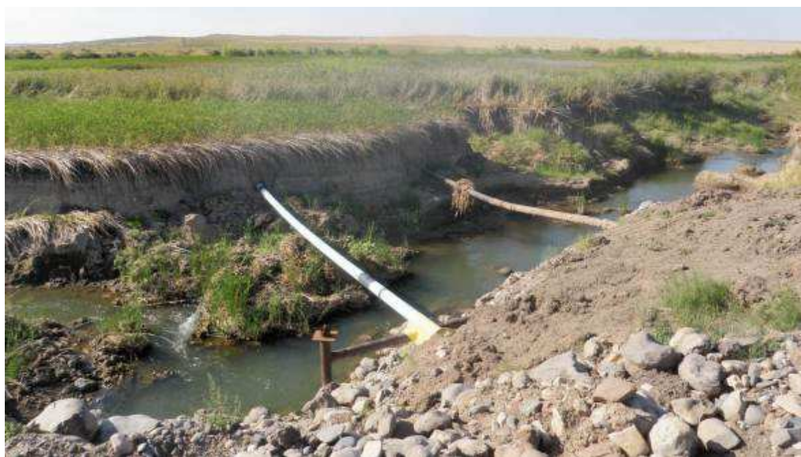
Conoco Phillips Seminole Pipeline at Beauvais Creek (Remediated)
